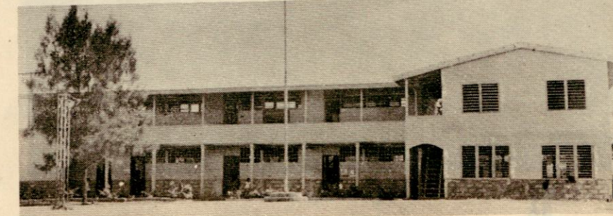
Camp Crame Elementary School (Pre-fabricated building)
